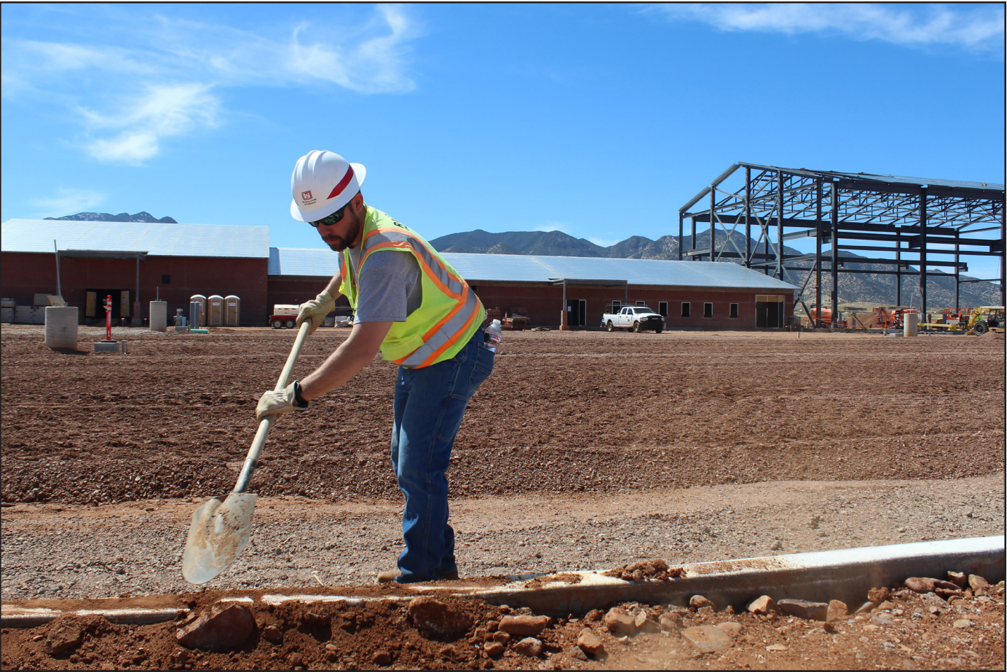
Contractor Thane Mir, a project manager with Rasch Construction Inc., removes sand and rocks from the curb before laying of pavement begins at the U.S. Army Corps of Engineers Los Angeles District’s Ground Transport Equipment project site March 14 near Sierra Vista, Arizona. Mir graduated from Colorado State University with a degree in construction management.
