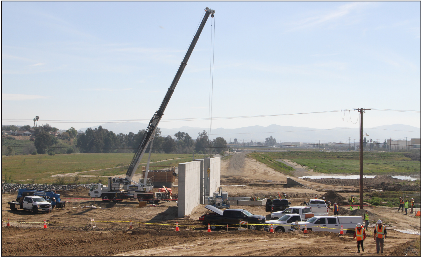
A crane is prepped before the installation of a 19-ton floodgate March 10 on the Alcoa Dike, alongside the Temescal Wash in Corona, California.
