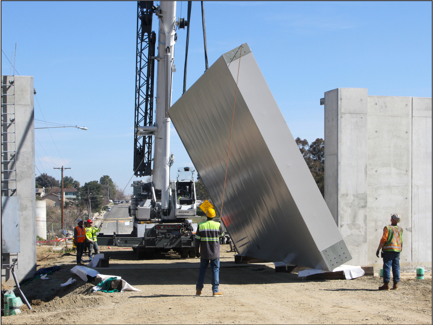
Contractors install a 19-ton floodgate March 10 on the Alcoa Dike, alongside the Temescal Wash in Corona, California.
