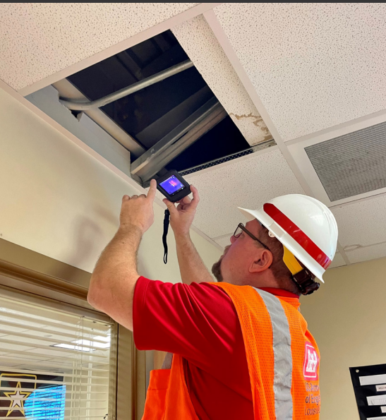
Tim McClellan, Louisville District National Roofing Program technical manager, inspects the roof at the Cape Coral Reserve Center in Cape Coral, Florida. (USACE photo by Abby Korfhage)
