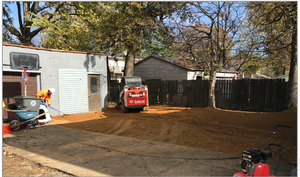
The U.S. Army Corps of Engineers Louisville District, in coordination with the Environmental Protection Agency, replaces contaminated soil with clean soil at a residential property, Nov. 9, 2022 in Evansville, Indiana. The remediation was prioritized by the EPA when high concentrations of lead were identified in a soil sample.
