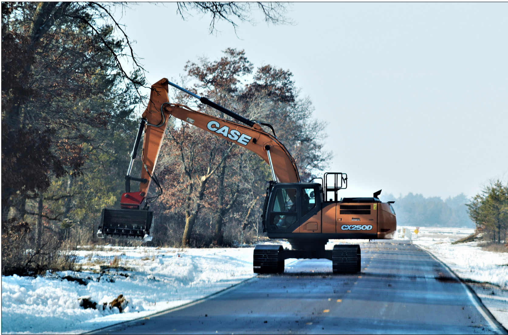
Fort McCoy Land Rehabilitation and Maintenance crew member Kris Steinhoff operates an excavator with a special attachment Jan. 11 along a roadway on South Post at Fort McCoy.
