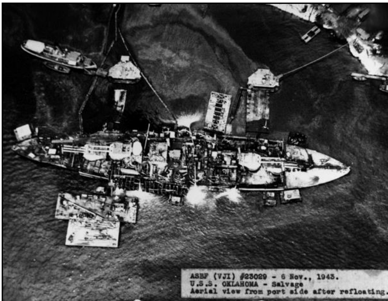
Aerial view from off the port side, Nov. 6, 1943, after the ship had been refloated. Note the large cofferdam patch installed from frames 43 to 75 to seal the extensive torpedo damage in that area, and cofferdams built around the main deck edge by the after turrets to increase the waterplane area and improve stability during the refloating process. Official U.S. Navy Photograph, from the collections of the Naval History and Heritage Command.
