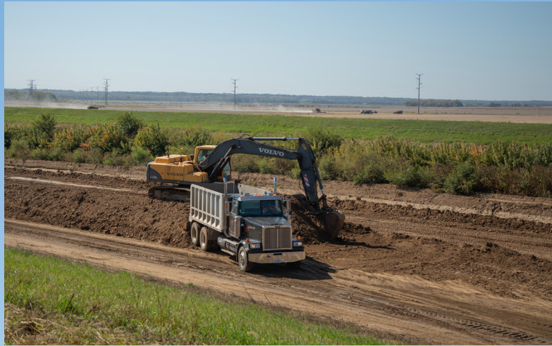
Contract employees excavate soil from nearby creek bed for rehabilitation of the Coal Creek Levee. Photo by Kelcy Hanson
