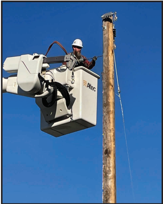
Steven Smith with Pine Bluff Arsenal's Directorate of Public Works, Electric Shop, reroutes power lines in compliance with lightning protection.
