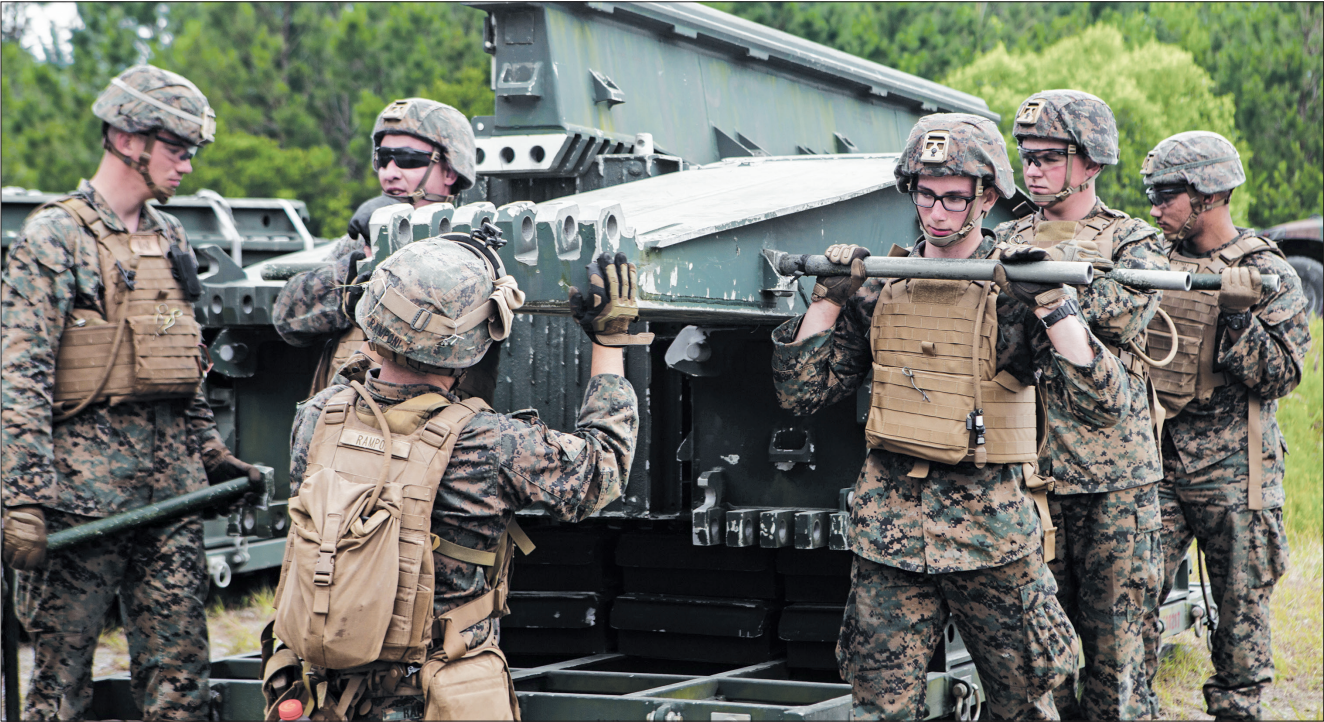
U.S. Marines with Bridge Company, 8th Engineer Support Battalion (ESB), 2nd Marine Logistics Group, assemble a medium girder bridge and improved ribbon bridge.
