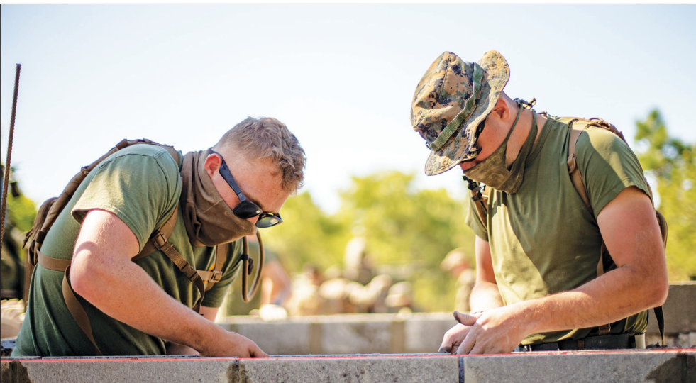
Lance Cpl. Mathew Dieter, left, and Cpl. Talon Malone, both combat engineers with SPMAGTF-SC, level a cylinder block wall. These training events provide the Marines and Sailors with real-world scenarios to prepare them for their deployment to Latin America and the Caribbean.
