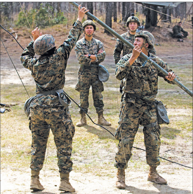
U.S. Marines erect an OE-254 radio antenna.
