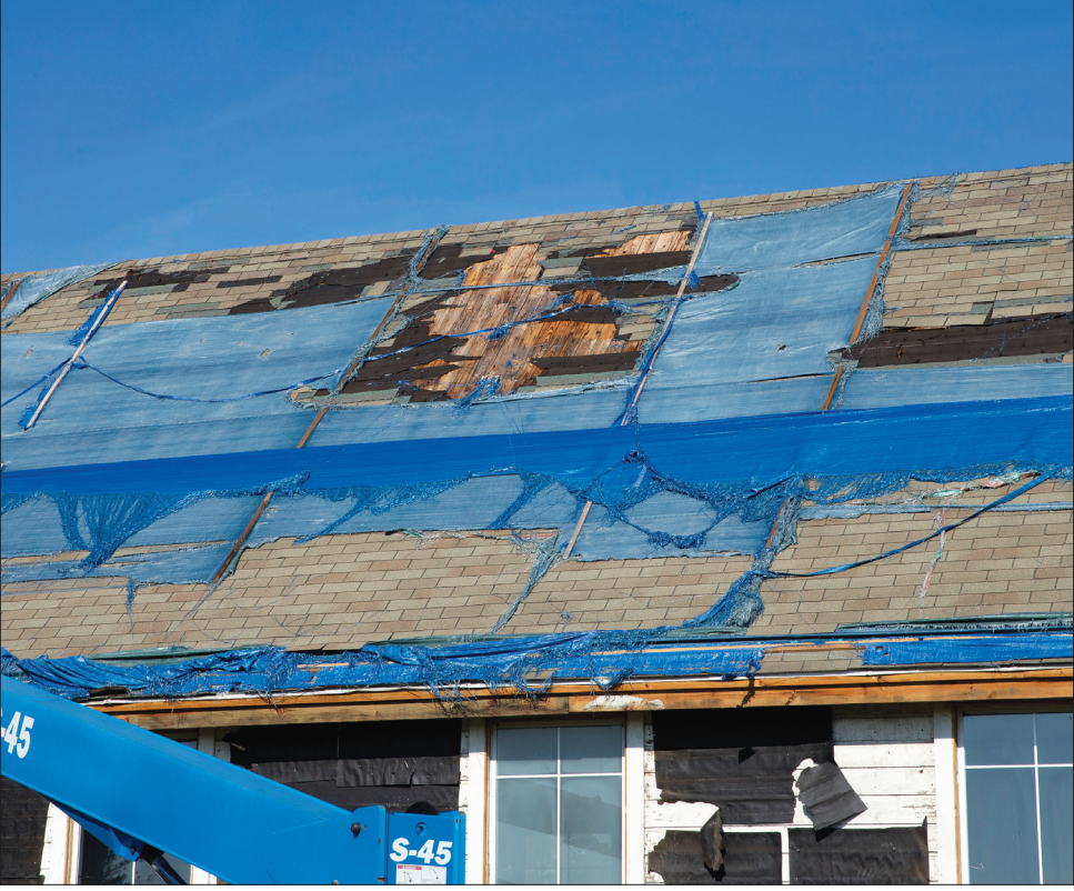
Structural damage to large portions of the roof are visible from the chapel exterior.
