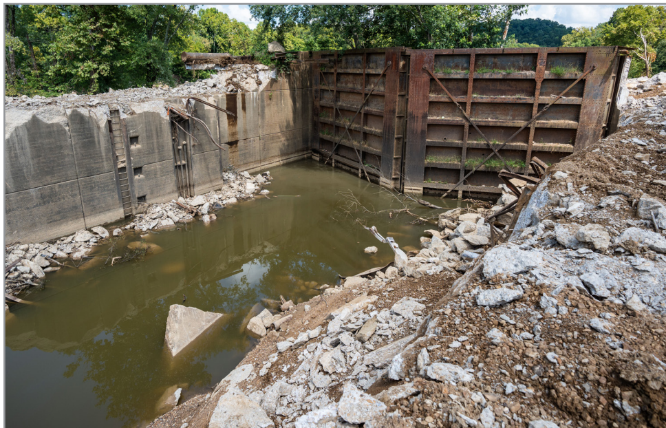
Barren River Lock and Dam 1’s structure, originally built in 1841 by the Commonwealth of Kentucky for commercial use, had deteriorated and was in an active state of failure. Federal legislation, under the Water Infrastructure Improvements for the Nation Act, was signed into law in 2016 deauthorizing the lock and dam site from the USACE inventory and directing its removal.
