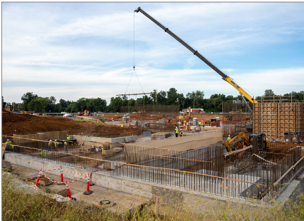
Contractors work on what will be the base of elevator shafts for the Louisville VA Medical Center, in Louisville, Kentucky, Sept. 2, 2022. Construction of the facility is anticipated to be completed in 2026.
