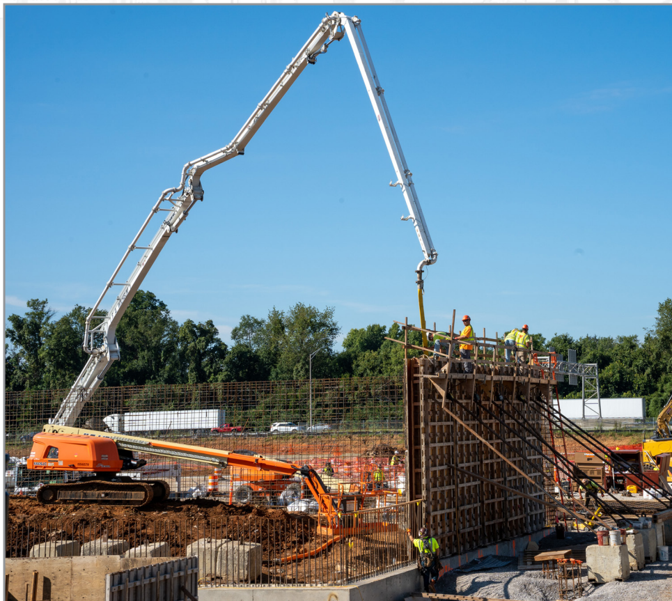
Contractors continue to place concrete sections of the basement walls of the Louisville VA Medical Center, in Louisville, Kentucky, Sept. 9, 2022.
