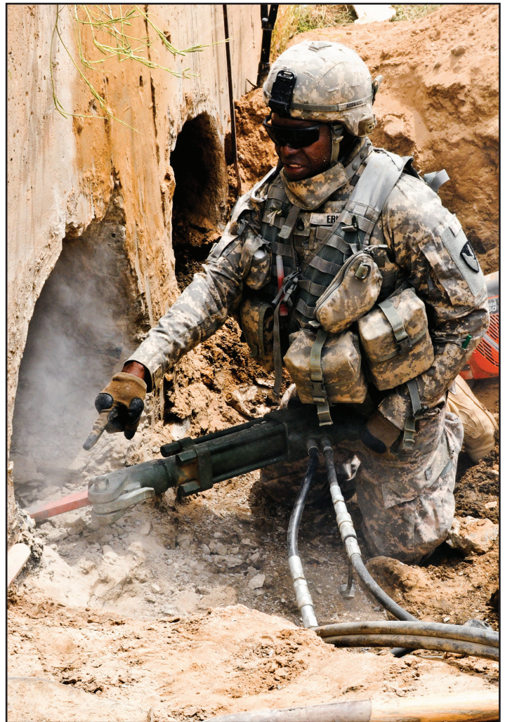
Photo by Sgt. Chad Nelson, 135th Mobile Public Affairs Det. Staff Sergeant James Eric, 3rd Plt., 573rd Clearance Co., 1st Eng. Bn., 130th Eng. Bde., uses a jackhammer to loosen up the concrete in a culvert. The engineers attempted to make the culvert's opening larger so they could install a "Lapeer kit," which is faster and more efficient than creating a metal grate.
