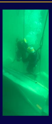
A 77,000-pound lift bag was suspended directly above the vessel, with two 10-ton chain falls attached to the lift bag's bottom by a strong back. ND2 Cayman Conley and ND2 Owen Craffey installed two 6,500-pound lift bags, one forward and one aft, to reduce overall weight and increase mechanical advantage for the Salvors to right the tug vertically for a much safer and more controlled lift.
