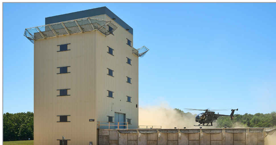
A MH-6M Little Bird helicopter lands on the Multi-Use Helicopter Trainer during a flight test at Fort Campbell, Kentucky June 29, 2022. The $5 million facility incorporates sea vessel flight deck configuration to facilitate safe and realistic training for aircrews and ground operators prior to operating in a harsh over-water environment.
