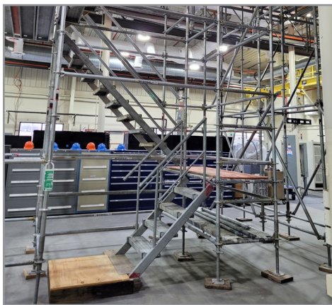
U.S. Army Corps of Engineers builds an elevated work platform to separate facility construction from the Submarine Battery Evaluation Center operation lab.
