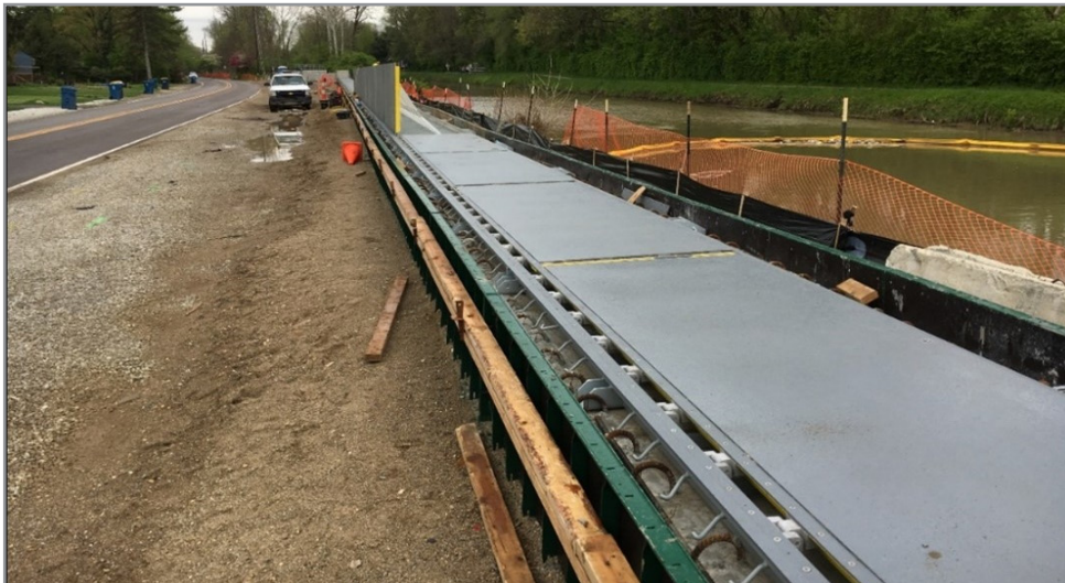
The innovative passive floodwall was constructed in 2019 is part of the Indianapolis North local flood protection project in Indianapolis, Indiana.
