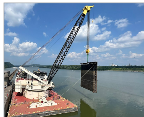
One of the old miter gates, weighing approximately 300 tons, at Cannelton Locks and Dam in Cannelton, Indiana, was removed July 23, 2022, marking a milestone in the five-month endeavor.
