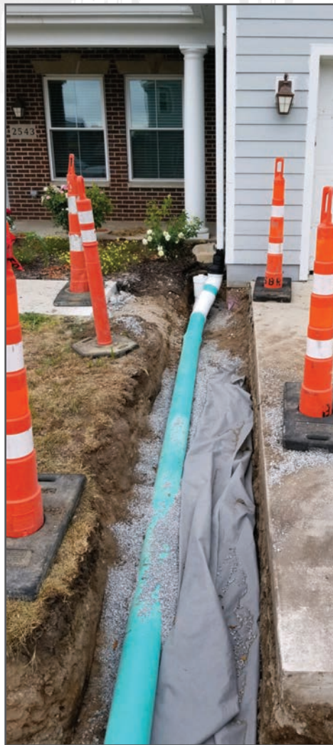
The Louisville District resolves the drainage issues at Rock Island Arsenal family housing area by designing a modification for a new underdrain system installation. The two photos above shows the work in progress (left) and then the completed project (right).
