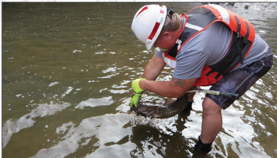
Keith Chaney, maintenance mechanic, helps remove debris and transfer fish and wildlife to outside the work area during the Clarence J. Brown Dam and Reservoir stilling basin dewatering event.
