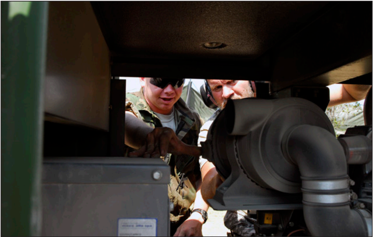
Sgt. William Valentine, generator mechanic, U.S. Army South, works with Victor Lopez, Department of Defense civilian contractor, on a new generator. The generator was having problems so they took off the frame to get a good look inside. (U.S. Army photo by Pvt. Cody Barber/11th PAD)
