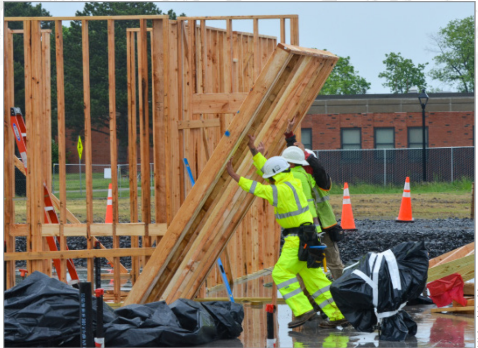
Contractors use teamwork to raise one of the walls of one set of cottages being built on the site of the Canandaigua VA Medical Center in New York. The cottages are part of Phase 2 of construction.
