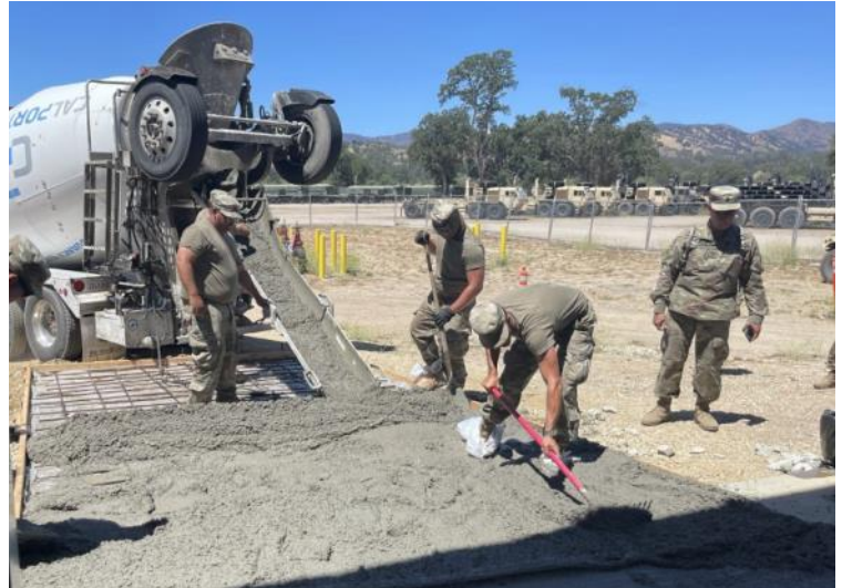
As part of their pre-deployment training, Army Reserve 471st Engineer Co. built a ramp for the TADSS Building allowing easier access for forklift operations to draw training aids and devices for units coming to train at FHL.
