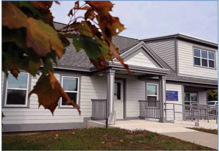
The “Cooper House” has been repurposed as the operations center of the NHNG Training Site in Center Strafford. The old 3,000-square-foot farmhouse was retrofitted with new windows, heavy spray foam insulation and heat pumps that enables it to run off just the solar electricity produced on site.
