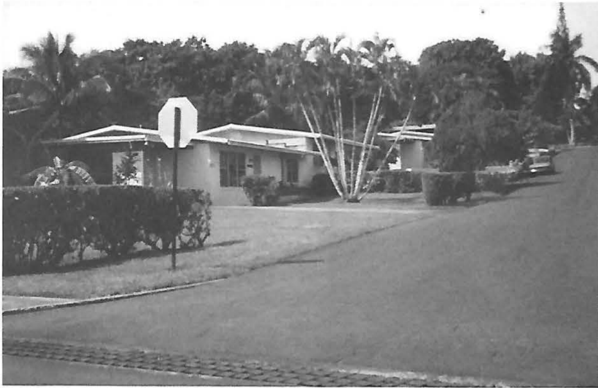
Thick jungle surrounds many of the U.S. housing areas in Panama. This aids the entry of trespassers or intruders into U.S. installations.
