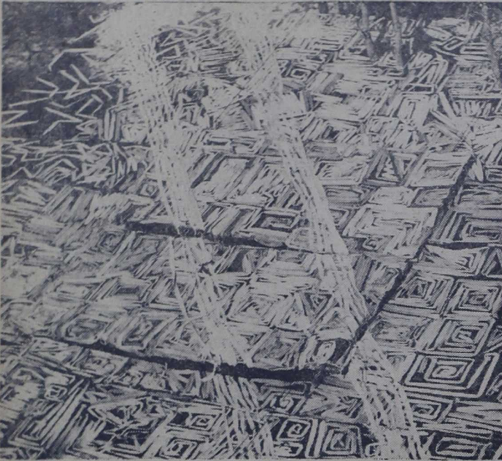
Guaranteed to drive Nipponese Aerial Photo Interpreters to saki is this camouflaged gun emplacement at the Engineer Battalion camouflage demonstration area. Note the blending of the dirt road and the net. From the air it looks like an ordinary dirt road.
