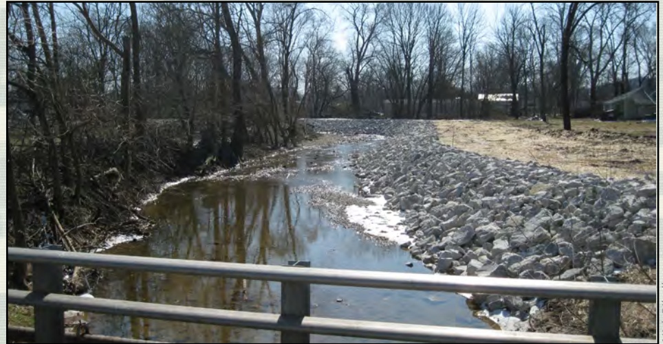
The Feather Creek channel was widened as part of a flood risk management project.
