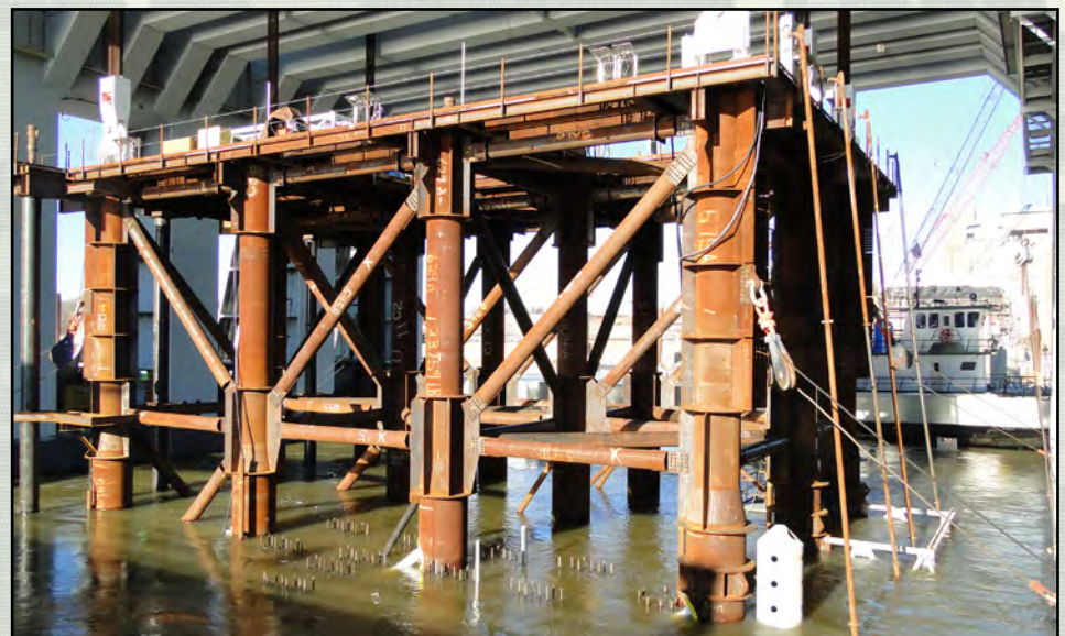
Still attached to the catamaran barge by the tubular lifting frame, Sill Shell No. 6 is lowered into place beneath the Ohio River Thanksgiving Day.
