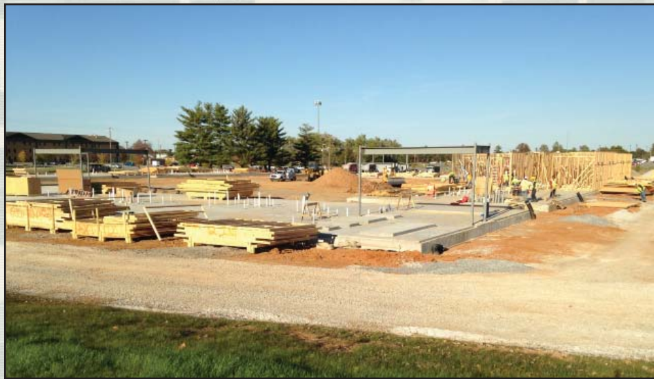
The steel structure and fabricated wood wall panels are going up on the new HHB Barracks, which will house Soldiers from the 101st Airborne Division at Fort Campbell.
