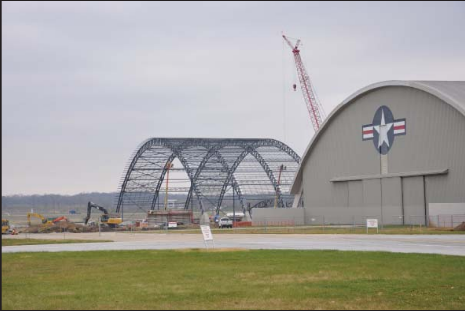
The structure of the new fourth building of the National Air Force Museum mirrors the design of the three existing hangars.
