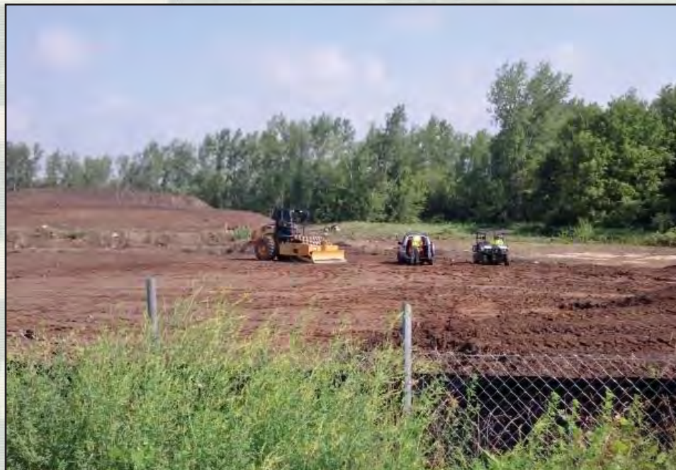
Contractors work to consolidate waste and create a soil cover at the Lockbourne landfill in Columbus, Ohio.
