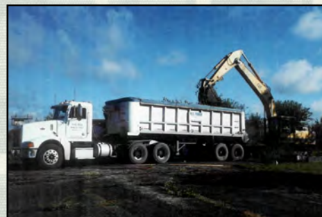
More than 485 cubic yards of soil containing polyaromatic hydrocarbons were excavated and hauled off the site to a Waste Management landfill.
