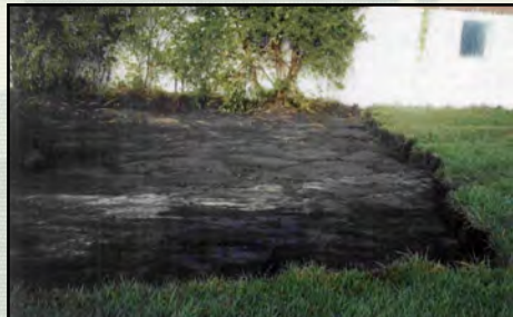
Twelve inches of surface soil was removed from the contaminated areas at the former Hanna City Air Force Station in Illinois and replaced with clean soil to restore the site.
