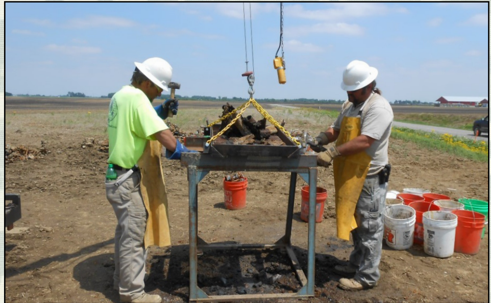
Site workers load the tray with munitions debris to be processed in the Thermal Flash Unit (TFU).
