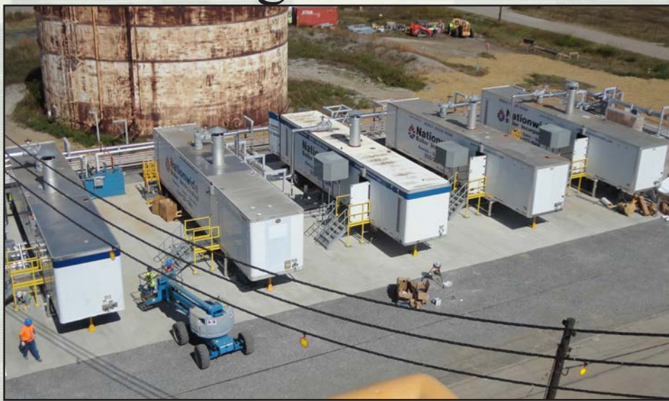
The new five steam package boiler units are shown at the Paducah Gaseous Diffusion Plant.
