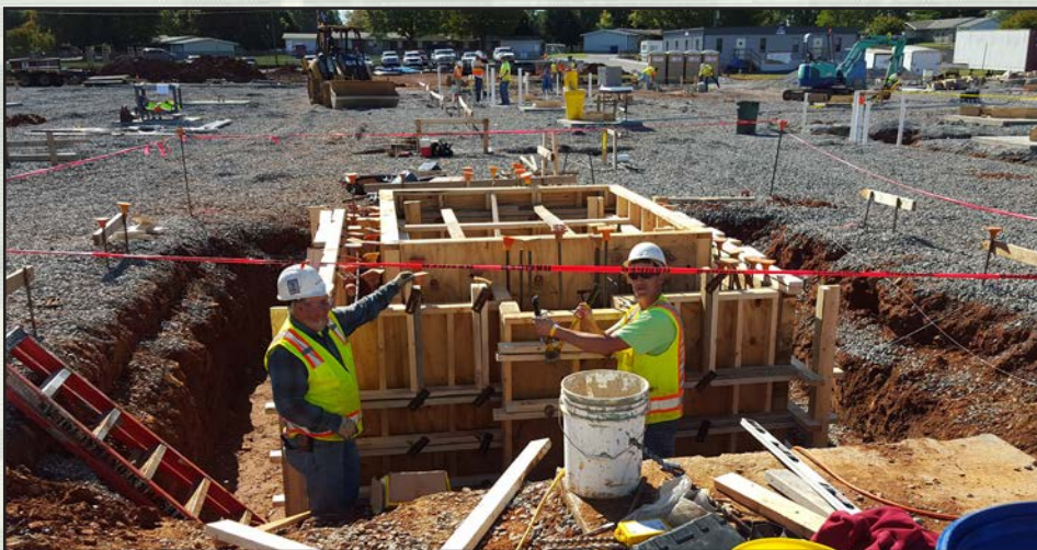
Contractors work on the forms for the vertical walls of the new school.
