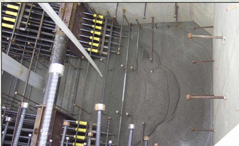
Self-consolidating concrete is poured into a lower pier shell at the Olmsted Dam Construction Project.
