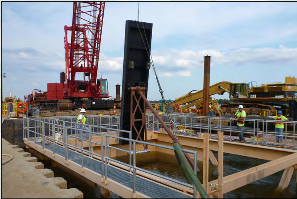
A new wicket is lowered by crane into the dive deflector box at Locks and Dam 53, which allows divers to replace deteriorating wickets while being protected from the strong flow of the Ohio River.
