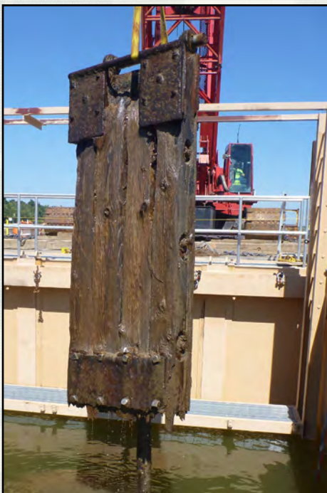
A deteriorated wicket is removed from the dam.
