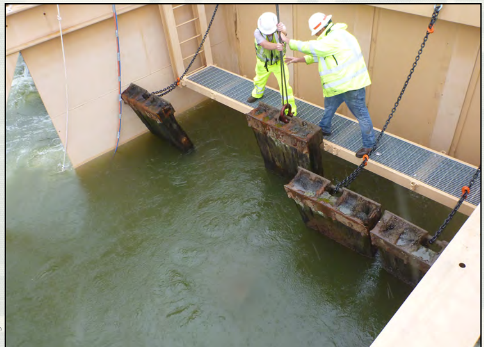
The rushing water of the Ohio River is diverted by the Dive Deflector box, creating a safe working environment for the crew at Locks and Dam 53 to remove old wickets from the dam.
