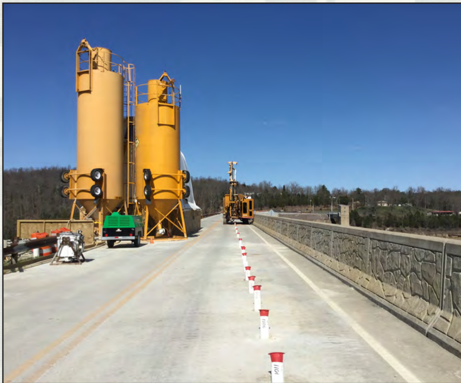
The concrete batch plant is in the foreground atop the Rough River Lake Dam, Ky. The white PVC casings are installed through the embankment to allow drilling and grouting in the rock foundation.
