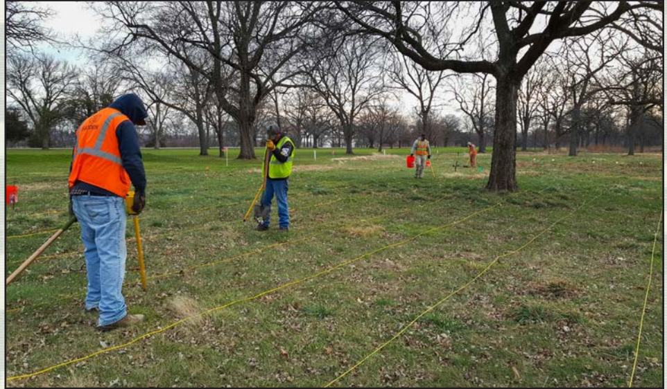
Contractors scan property at Rock Island Arsenal to detect metal objects up to a two-foot depth. In the thorough scan of more than four acres, contractors found two grenades.
