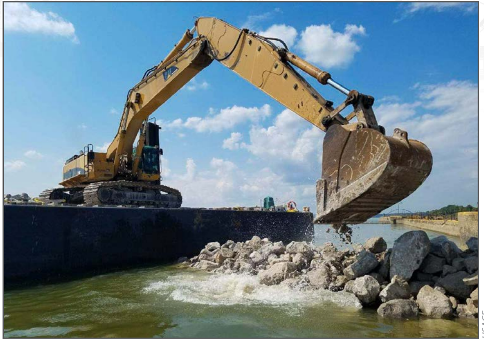
The Corps has built a rock dike, which will protect divers as they replace wickets in Dam 52.
