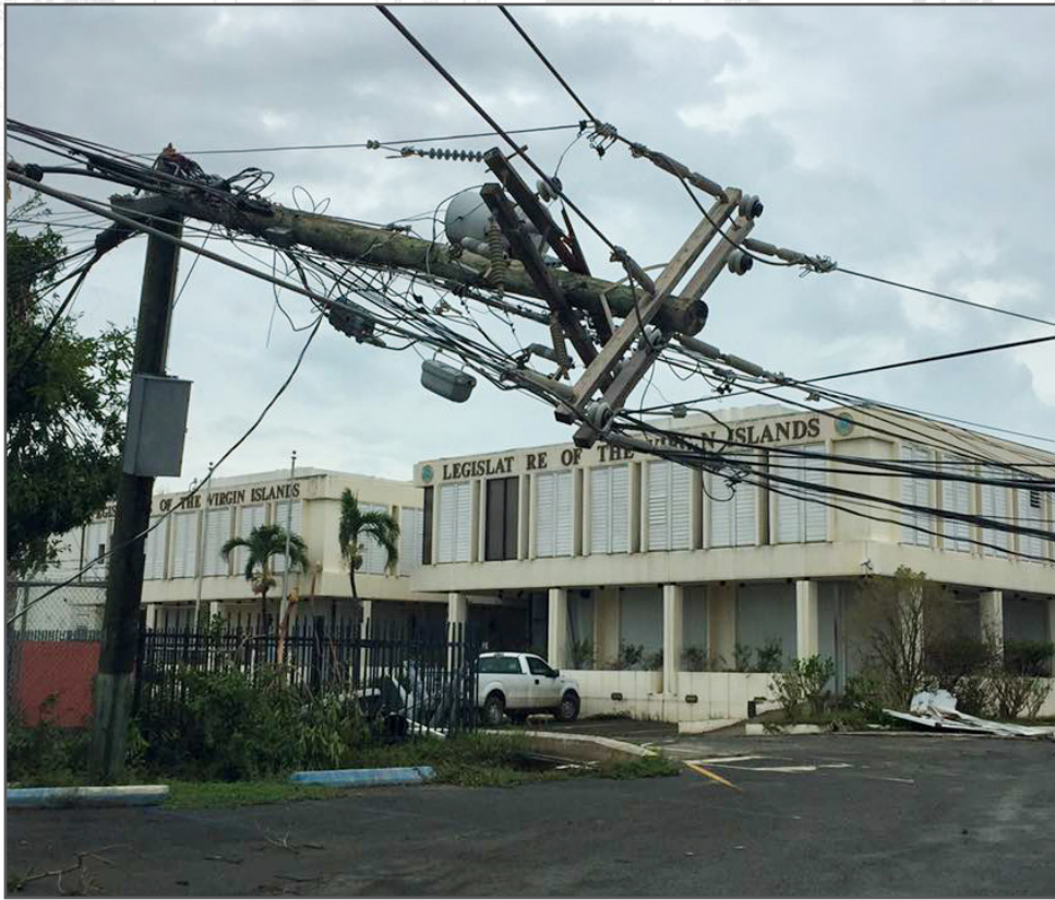
A telephone pole is snapped in two outside the Legislature of the Virgin Islands office building in Frederiksted on St. Croix, USVI.
