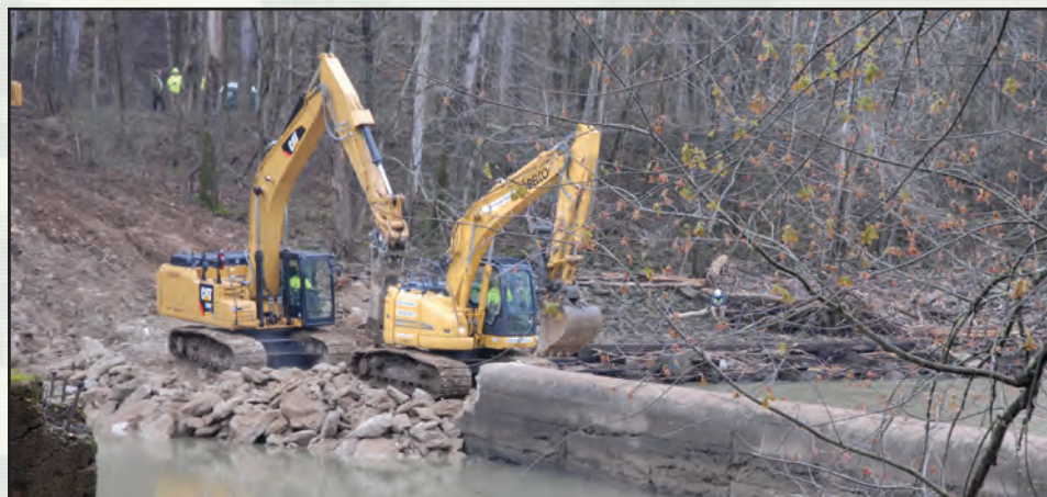
The excavators break up Dam No. 6 while building a work pad from which to remove material during the demolition, which was completed in April.
