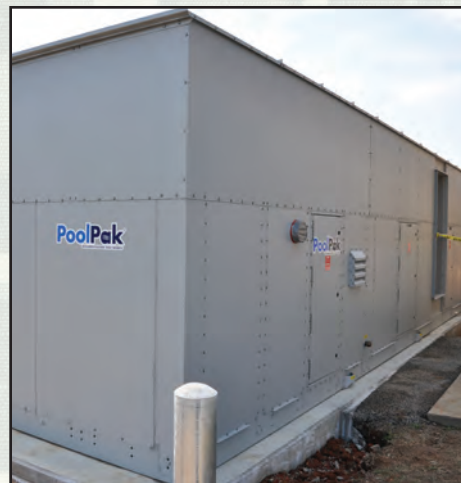
The new air handling unit has more capacity to properly dry the air and control the temperatures throughout the facility.
