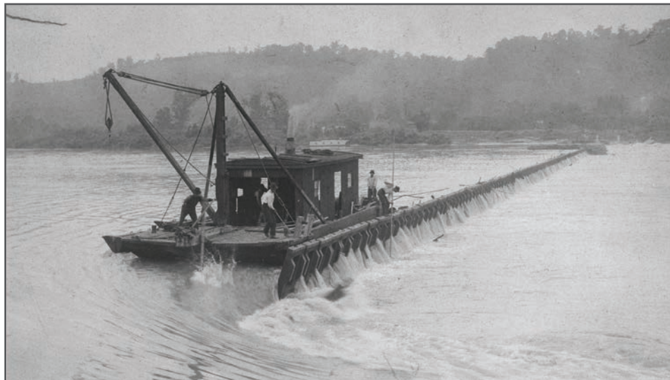
Historical photo of the wicket dam being raised at Lock 52 in Brookport, Ill.
