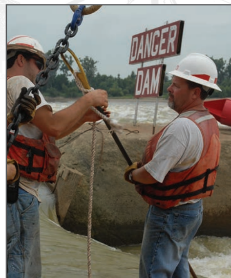
USACE employees work together to raise the wickets in 2011 at Locks and Dam 52 in Brookport, Ill.
