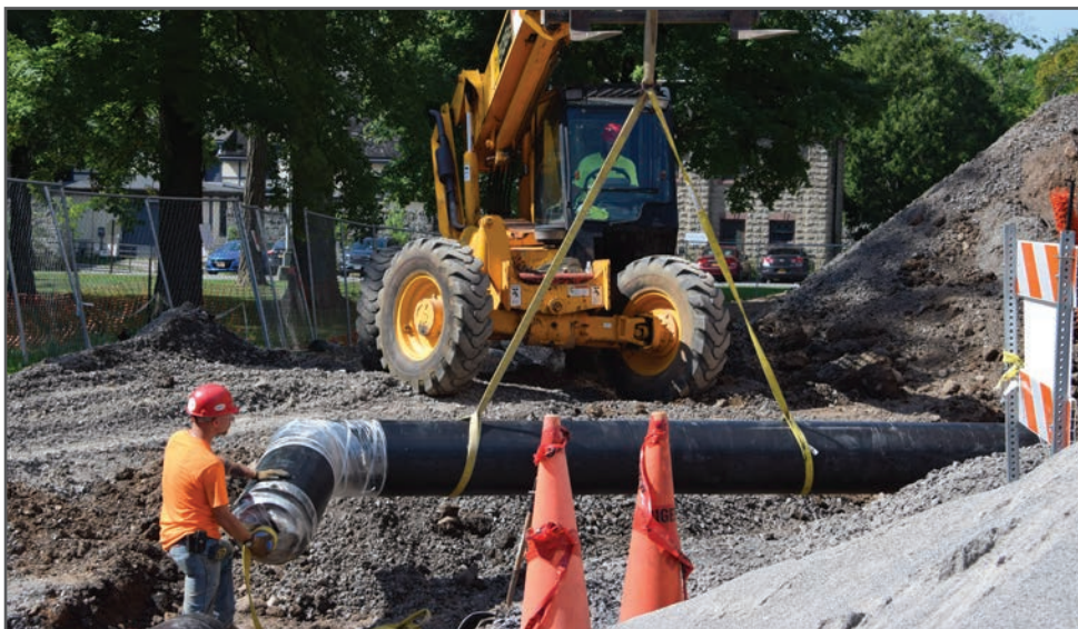
Personnel continue construction at Canandaigua VA Medical Center Sept. 4, 2018.
