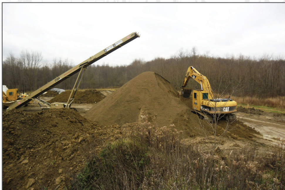
Up-armored excavator moves sifted soils for final munitions clearance prior to shipment for off-site disposal during the latest remedial action at Winklepeck Burning Grounds at the former Ravenna Army Ammunition Plant in Ohio.
