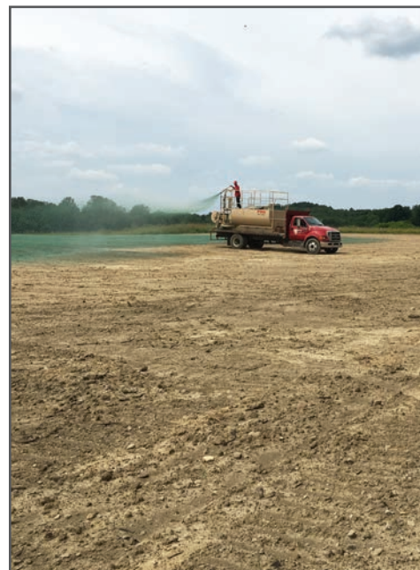
Excavation sites were graded and reseeded at the completion of the remedial action. A native seed mix was utilized at each excavation site for reseeded.
