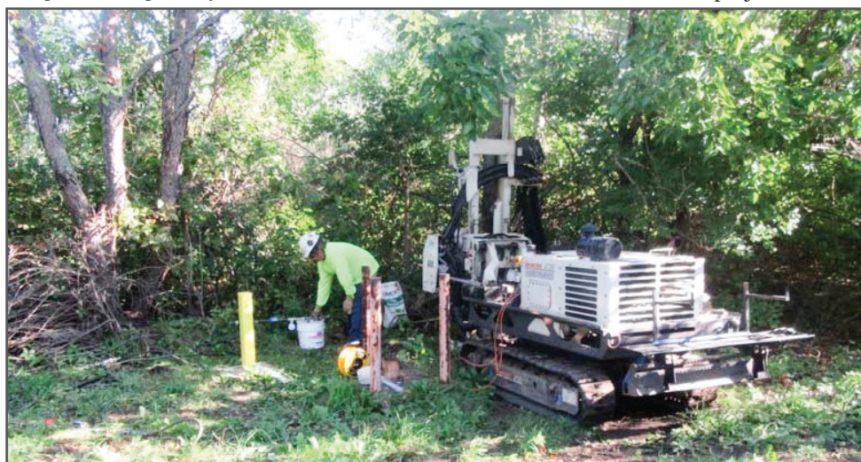
A contract worker observes the injection system inserting material into the subsurface of IP-3 in the northeast corner of the injection area at former Nike C-47.
