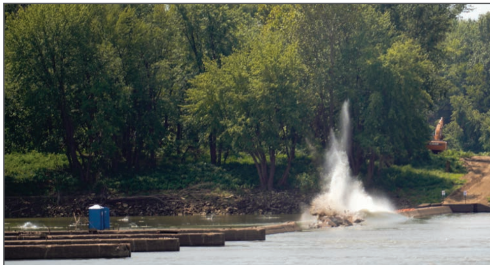
Ohio River Locks and Dam 52 Fixed Weir demolition took place Aug. 21, 2019. With the completion of Olmsted Locks and Dam the concrete demolition of LD 52 begins with the explosion of the fixed weir on the Kentucky side of the river.
