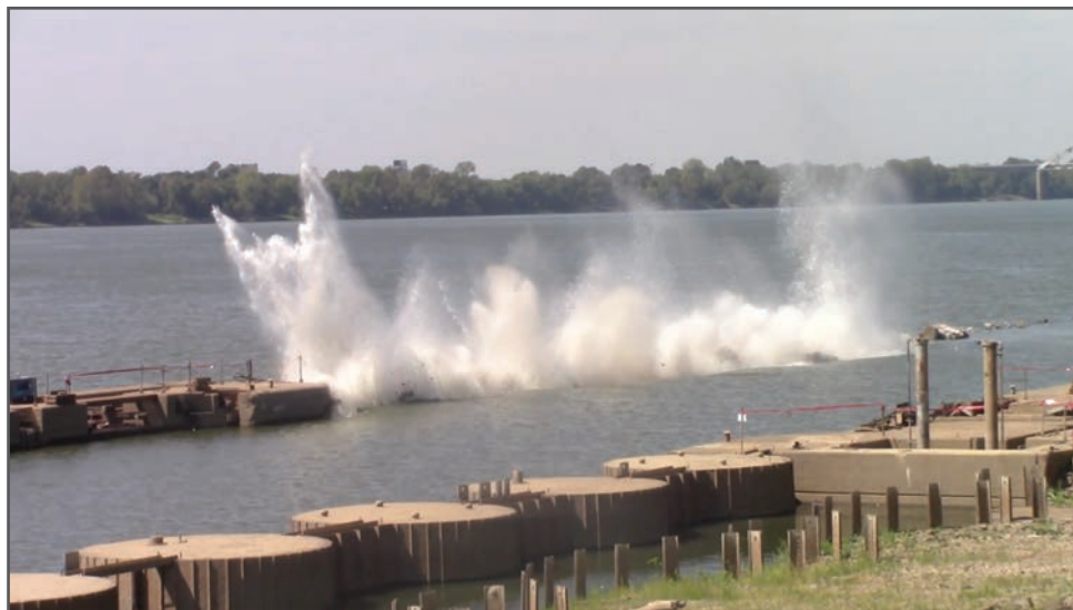
Demolition of Lock and Dam 52 in Brookport, Illinois, began Aug. 8, 2019. The demolition is being completed using blasting methods to fracture portions of the concrete structure to break it up for easier removal with heavy machinery.
