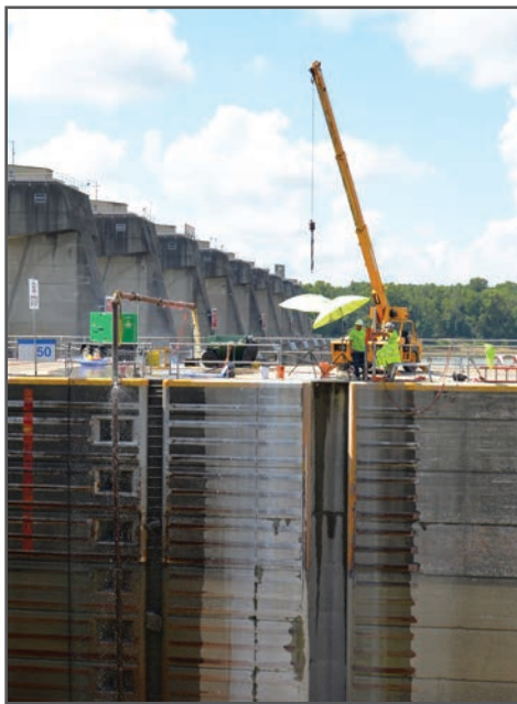
Contractors perform core drilling to replace floating mooring bitt tracks in the main chamber at John T. Myers Locks and Dam Aug. 18.
