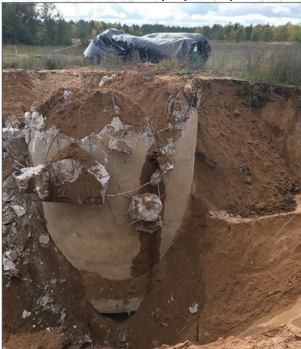
During the field investigation at the Raco Army Airfield and Missile site in 2016, a partially demolished settling tank filled with TCE (trichloroethene) contaminated sludge, 18 feet in depth, was discovered. Prior to the completion of the Non-Time Critical Removal Action to remove the tank, approximately 61 tons of concrete and 104 tons of soil/sludge remained in Vault 4.
