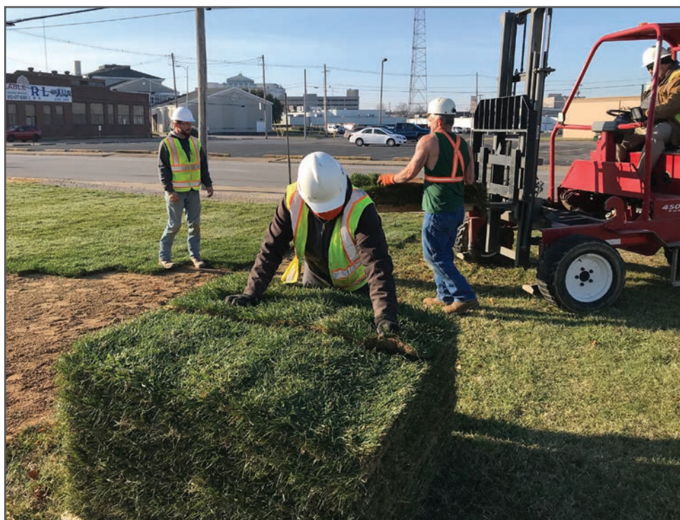
Contract workers install clean sod, consisting mostly of fescue and some with zoysia, at residential properties of the Jacobsville Neighborhood Soil Contamination Superfund site.
