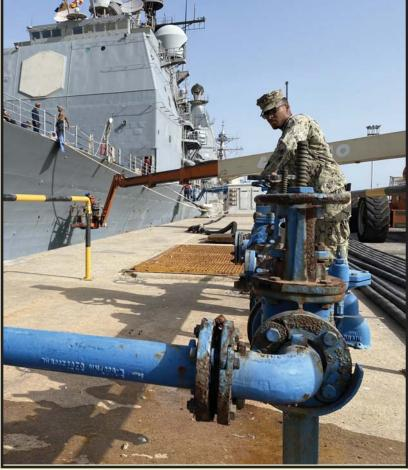
UT2(SCW) Wilson from UEM Water distribution branch is down at Pier 1 hooking up one of the DDGs with potable fresh water. Just like shore power connections, the water directly allows the ship to run normally and with less watch standers once NAVFAC hooks them up! UEM's water crew is responsible for the water connections for each individual ship down Pier 1, along with monitoring water and waste water usage.
