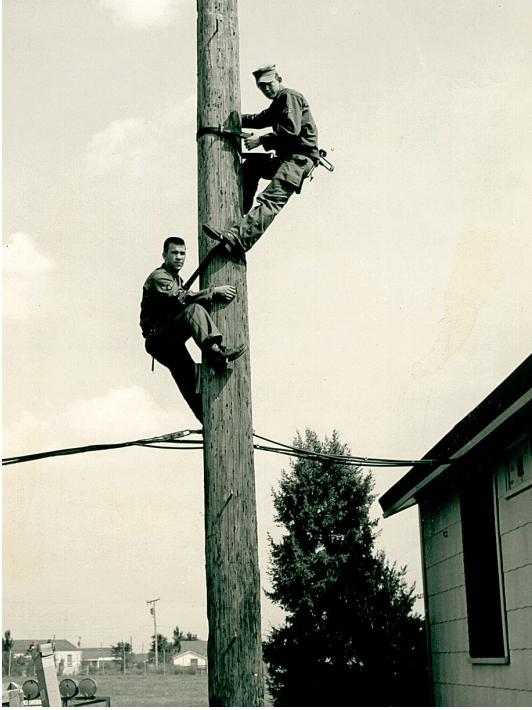
Installers use climbing gaffs to climb a telephone pole to install communications cables.
