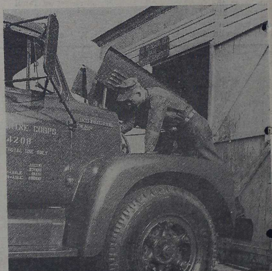
WINTERIZING —Pfc Bruce W. Knowles, a mechanic for the First Platoon, checks the water hose on one of the platoon's vehicles while winterizing them for the coming winter months. All water hoses must be checked and old ones replaced before filling with antifreeze.
