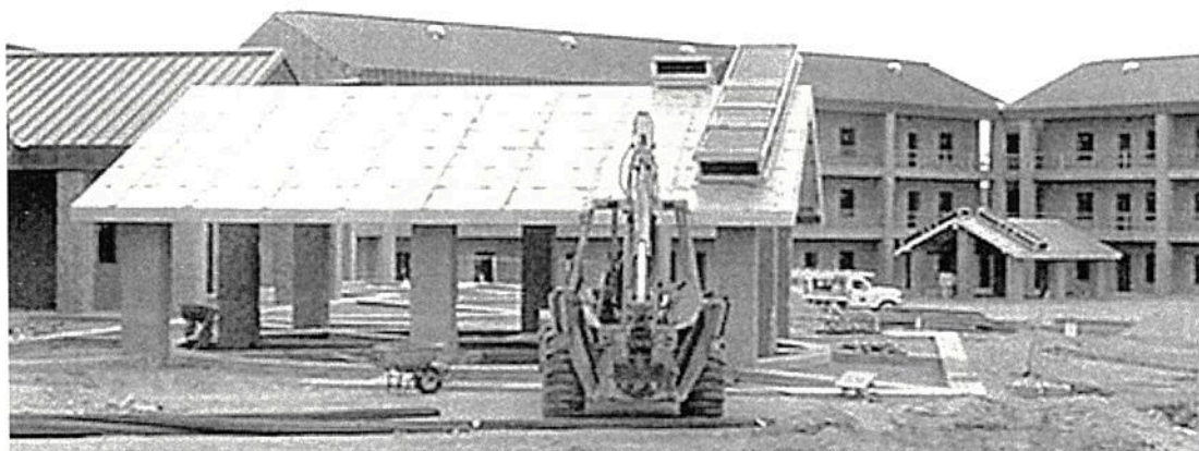
New barracks central area under construction at Fort Irwin.
