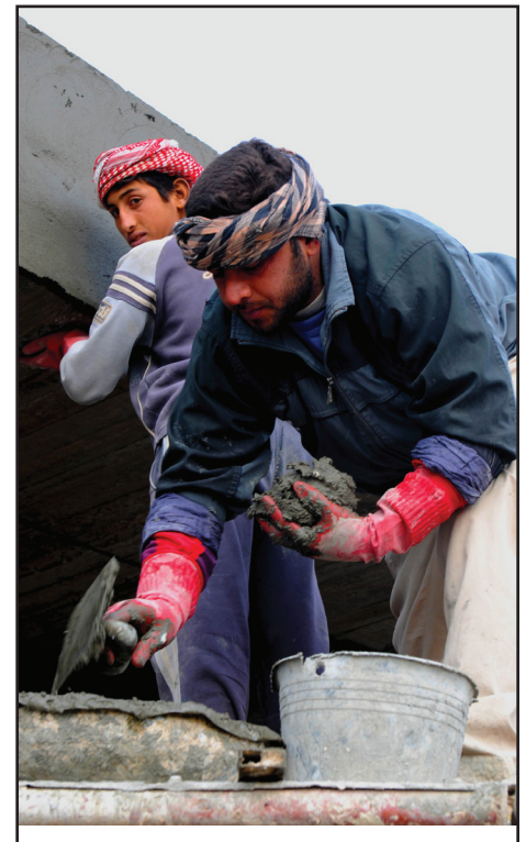
Photo by Sgt. Chad Nelson, 135th Mobile Public Affairs Det. A worker with Brother Group Construction and Services gathers concrete to lay on the façade of a new school being built in Al Khanag village.
