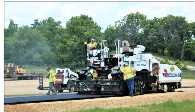
Contractors put down pavement June 2, 2021, on a road near Pine View Campground at Fort McCoy. The work is part of many types of roadwork taking place in 2021.
