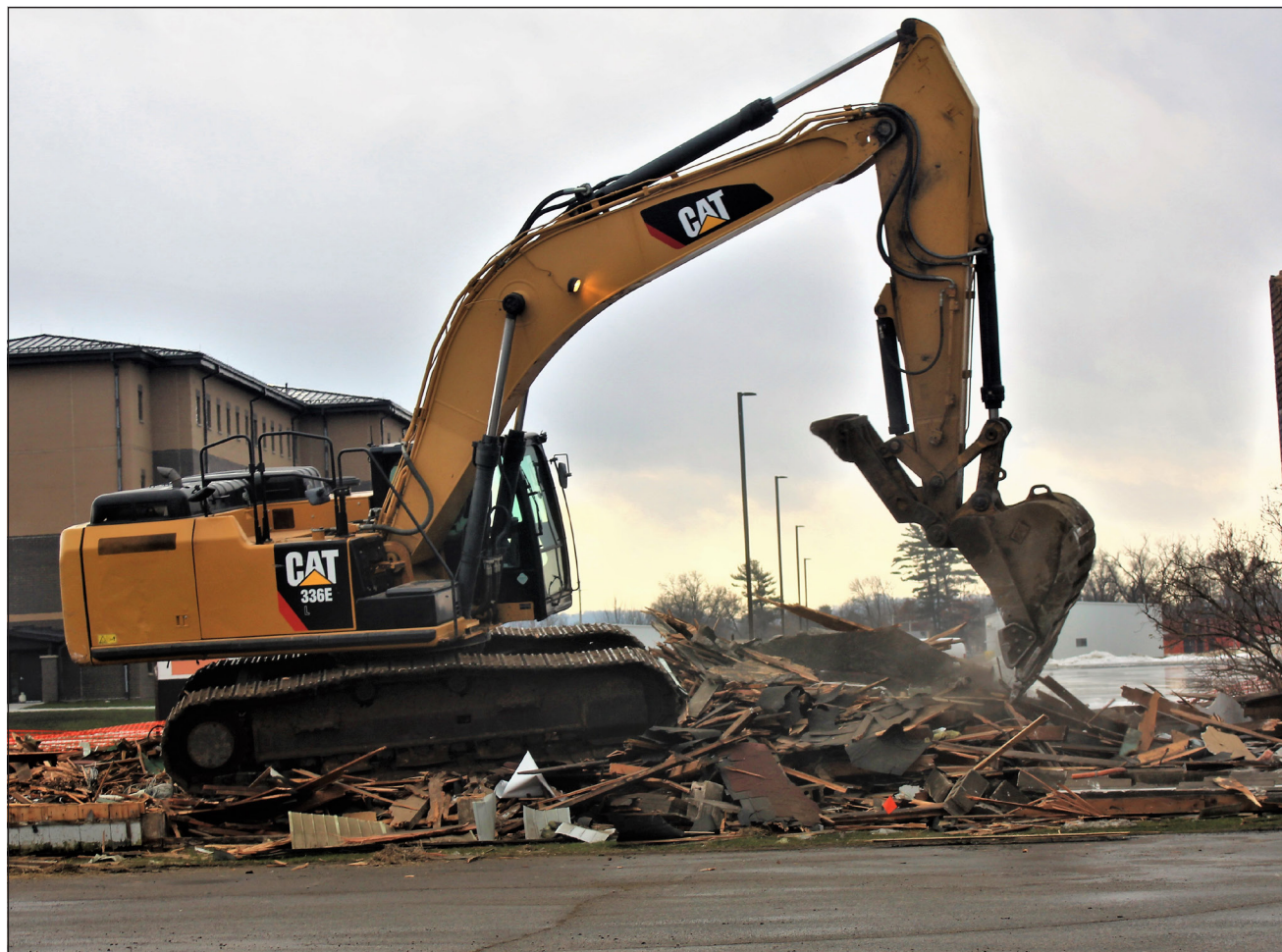
A worker uses an excavator to take down a building in the 1600 block of the cantonment area Dec. 15, 2021, at Fort McCoy. The work was to make way for more construction in 2022 for the first of three new brigade headquarters buildings.
