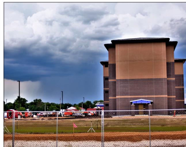
Storm clouds move over Fort McCoy on June 11, 2021, while ongoing construction on the first new barracks building project is shown.
