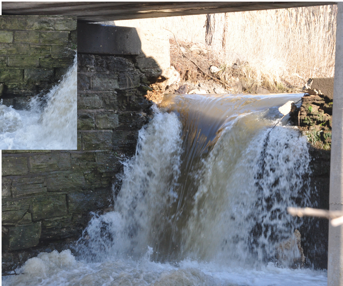
Above, the bridge abutment shows signs of failure. Right, Blackberry Creek flows through the notch placed in the dam to start mitigation for the eventual removal of the dam and replacement of the bridge.
