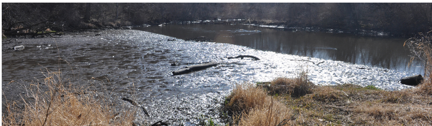
Floodplain benches above the dam on Blackberry Creek became exposed after the water level dropped following the notching of the dam.
