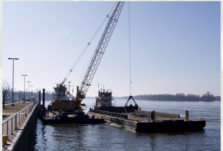
Mississippi River Project mechanical dredge crews work to remove material along the upper approach wall to Lock and Dam 17 this spring.
