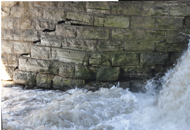
Above, the bridge abutment shows signs of failure. Right, Blackberry Creek flows through the notch placed in the dam to start mitigation for the eventual removal of the dam and replacement of the bridge.
