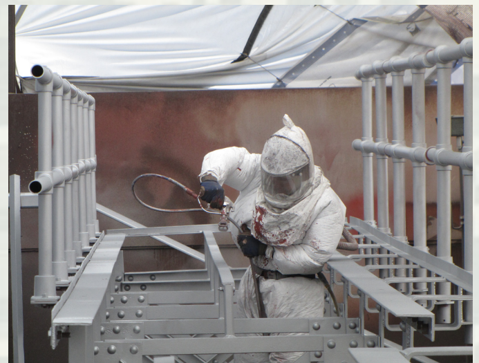
Tim Scranton, Mississippi River Project, paints the #2 miter gate walkway from Lock and Dam 17 at the Mississippi River Project Service Base. The refurbished miter gates are scheduled to be reinstalled in June.
