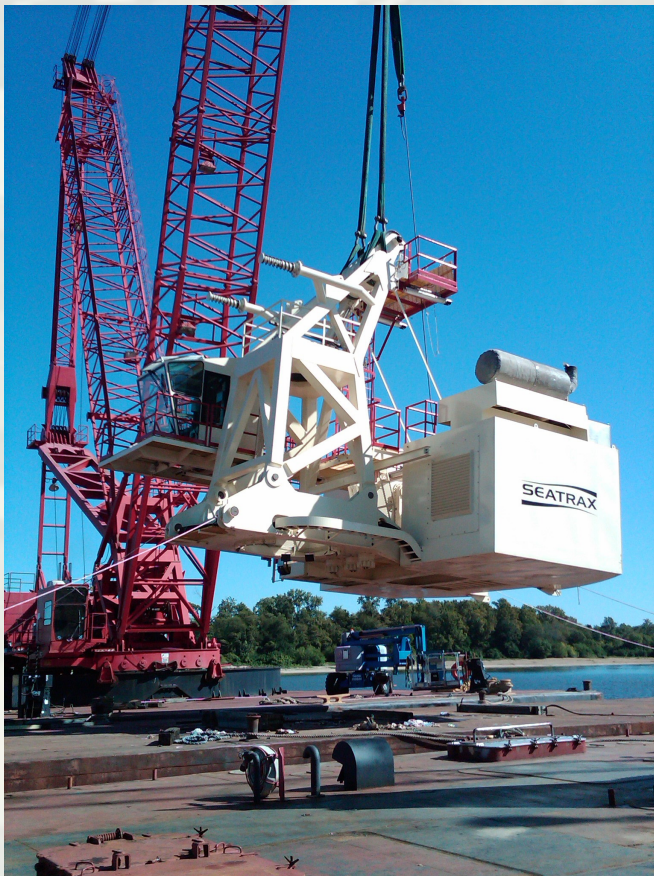
The Illinois Waterway Structures Maintenance Unit's heavy-lift crane Hercules helped place the new Seatrax Crane onto its pedestal at Ensley Engineer Yard in the Memphis District.
