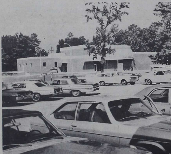
READY FOR OCCUPANCY — The new Marine Exchange service building located next to the Main Exchange will be ready for use this week. Built by the Dixie General Construction Company of Wallace, N.C., the building was officially accepted by Base officials this month.
