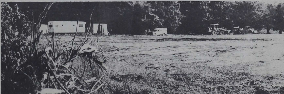
FIRST STEP — An empty field is all one sees of the new Hostess House which will be built next to the bank on Holcomb Blvd. Members of Danlee Construction Company, Jacksonville, Fla.,
