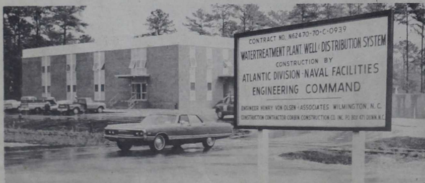
WATER WORKS — The new Water Treatment Plant, well and distribution system here was recently accepted by the base and is now in full operation. The plant, located near the Main Gate off Holcomb Blvd., was built at a cost of $1.8 million.
