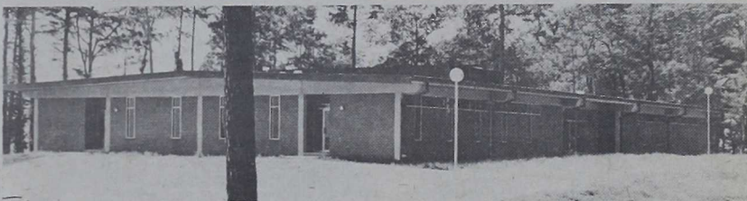
DENTAL BUILDING — The 2d Dental Company, 2d Marine Division, has been presented the new Dental Building located on River Road. Patients will soon be treated in early September in the new facility as soon as furniture and supplies are moved in and installed.
