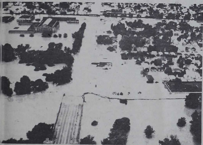
ROAD TO NOWHERE — A highway somewhere near Wilkes-Barre, Penn. abruptly ends, a victim of Tropical Storm Agnes. Because so many roads were washed out, everything from small boats to helicopters were used to carry the evacuation of stranded people. (U.S. Coast Guard Photo)
