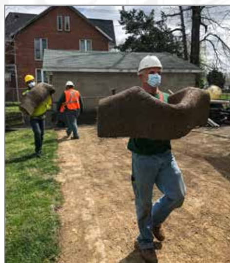
Workers install sod at a Jacobsville, Indiana residential property that is being remediated for contaminated soil, April 6, 2021. The U.S. Army Corps of Engineers, on behalf of the Environmental Protection Agency removed and disposed of 17,940 cubic yards or 23,322 tons of lead and arsenic-contaminated soil for the 2021 field season. Residences received 25,010 cubic yards of clean soil and 571,031 square feet of new sod.
